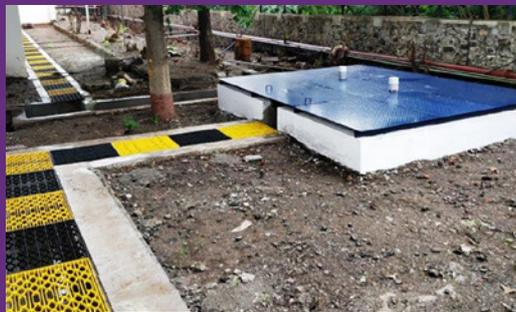
*The new rainwater collection and storage system is protected from evaporation losses.*
